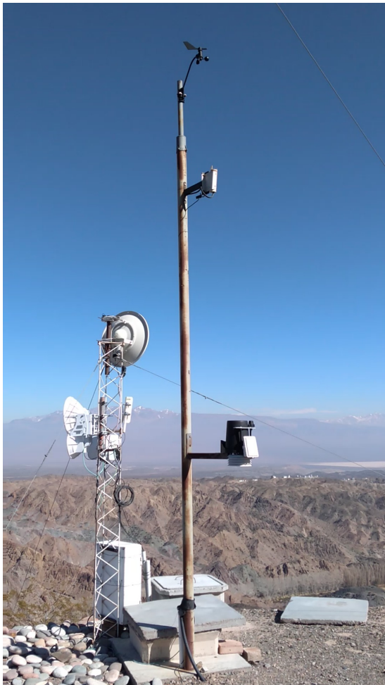
Figure 1: Sensors of the Davis Vantage Pro2 meteorological station installed at Cerro Burek.
